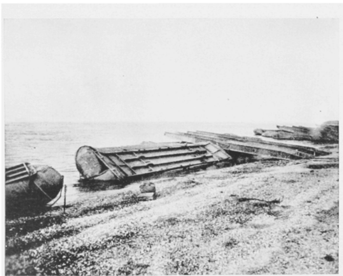
DAMAGED FLOATS CAUSED BY CLASS 40 BAILEY RAFT DRIFTING INTO M2 TREADWAY BRIDGE AT WALLACH
