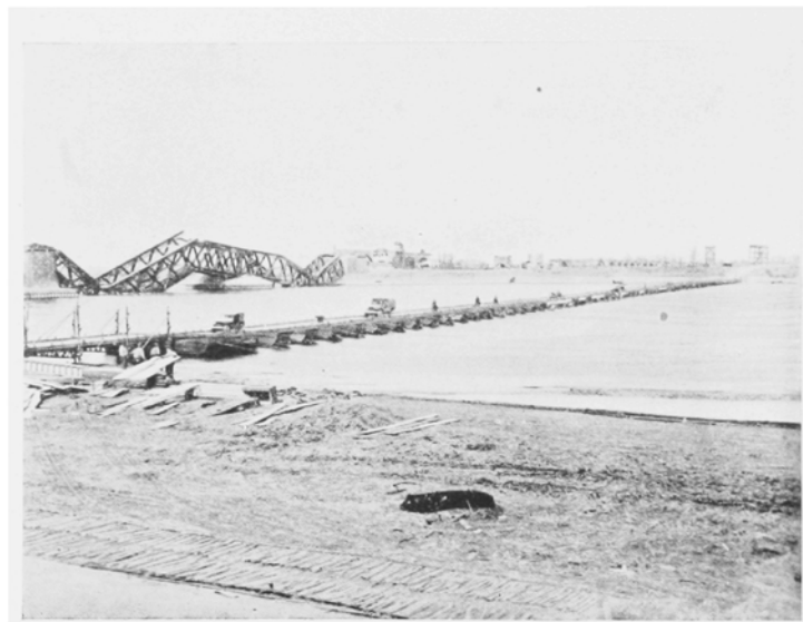
COMPLETED 25-TON BRIDGE CARRYING TRAFFIC AT WESEL
