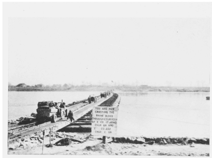
COMPLETED M2 TREADWAY BRIDGE AT WALLACH
