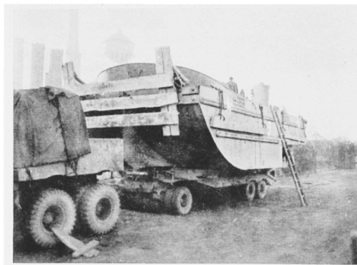
SEAMULE (COMPLETELY ASSEMBLED) LOADED ON MIQ TANK TRANSPORTER
