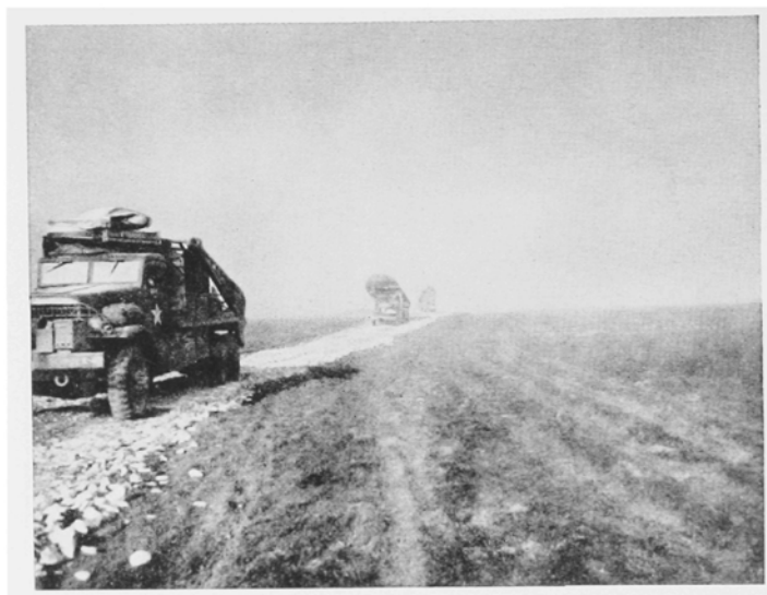
TRUCKS CARRYING TREADWAY BRIDGING ON APPROACH ROAD TO BRIDGE SITE AT WALLACH. THE ROAD WAS CONSTRUCTED OF SOMMERFELD TRACK COVERED WITH ROCK
