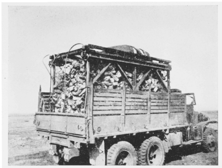
BAILEY CRIB ANCHOR TO BE USED ON MI TREADWAY BRIDGE AT MEHRUM
