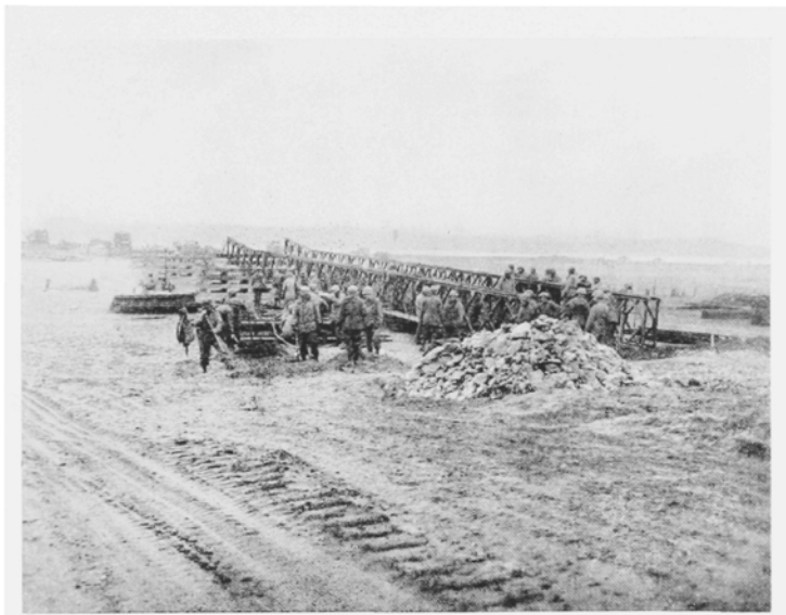
WEST SHORE FIXED SPAN UNDER CONSTRUCTION, BAILEY BRIDGE NO. 2
