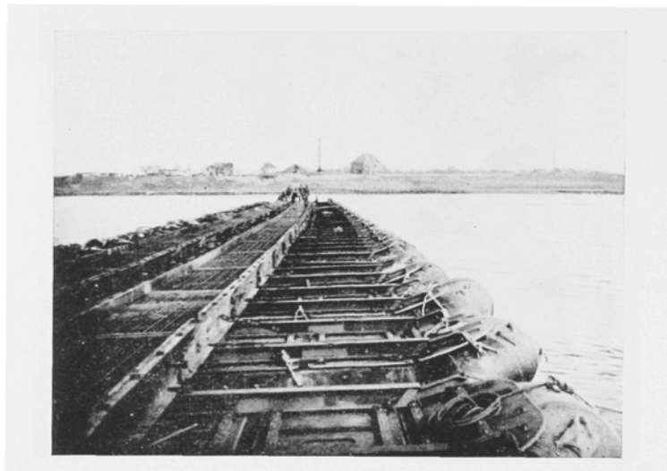
M2 TREADWAY BRIDGE AT MILCHPLATZ UNDER CONSTRUCTION
