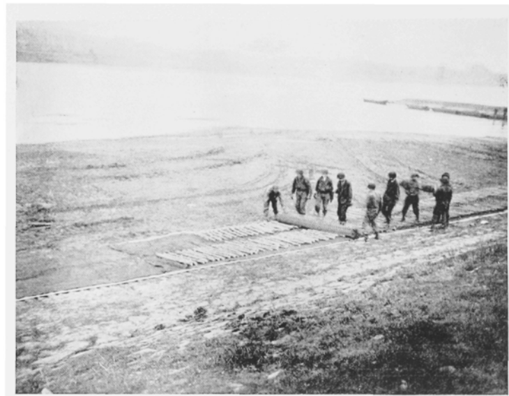
LAYING EXPEDIENT ROAD APPROACH TO THE WESEL BRIDGES
