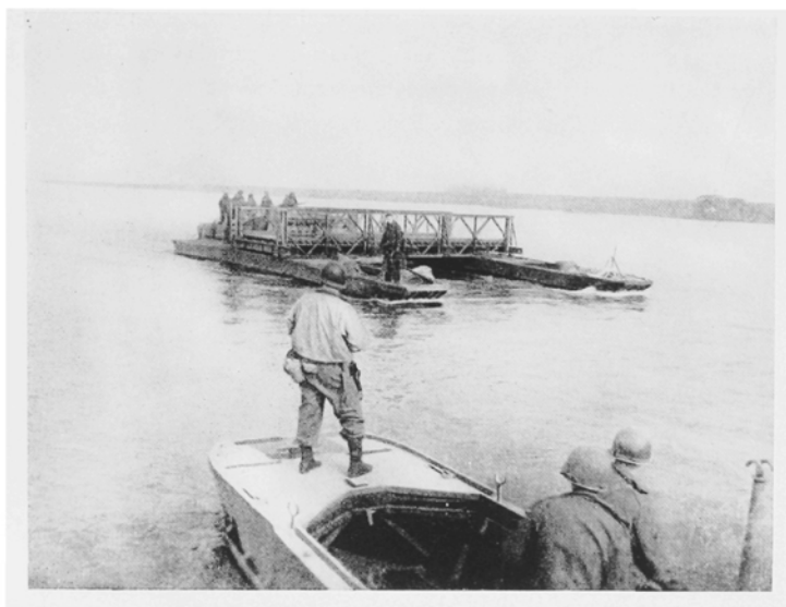
A FLOATING BAY BEING MOVED INTO PLACE, BAILEY BRIDGE NO. 2
