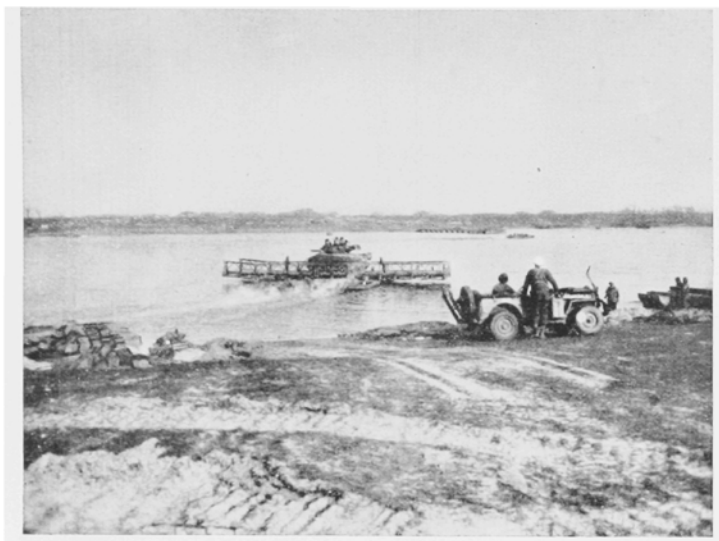
MEDIUM TANK BEING CARRIED TO FAR SHORE ON CLASS 40 BAILEY RAFT. OFFICER WEARING THE WHITE HELMET IS "BEACHMASTER"
