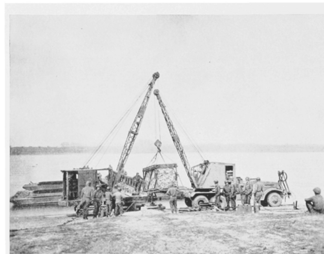
TWO CRANES LOADING A CRIB ANCHOR FOR BAILEY BRIDGE NO. 1 ON TO A BAILEY RAFT
