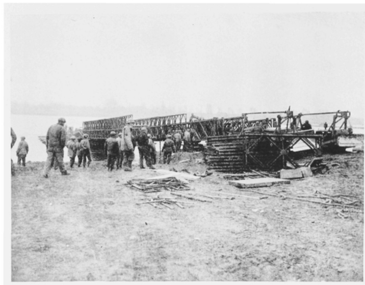
LAUNCHING THE WEST SHORE LANDING BAY, BAILEY BRIDGE NO. 2
